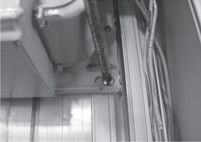
**Step 1** – Replace the screws holding the transformer in place using a Phillips head screwdriver (two point).
